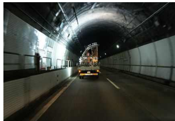
Figure2 The inspection situation by the picture photography technology
