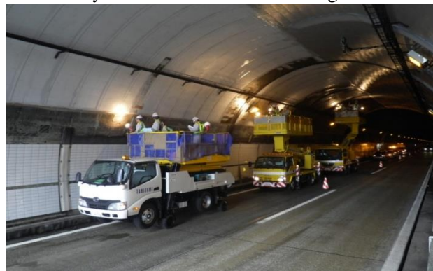
Figure 1 Approach watch/tapping sound inspection circumstances
